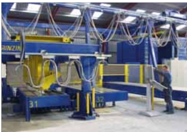
Automatic filling of system moulds with SCC
