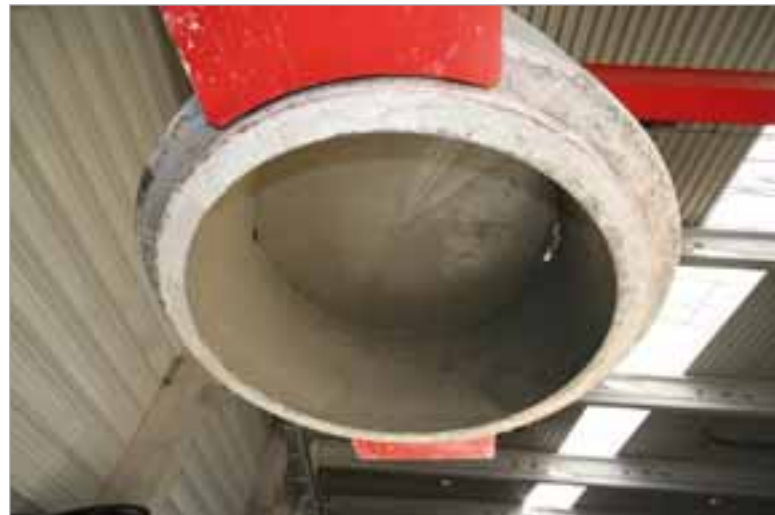
Monolith following removal of the inner support core
