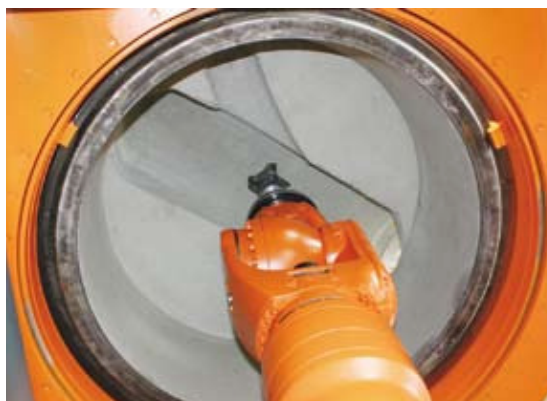
Fig. 6 The drains are milled out with pinpoint accuracy.
