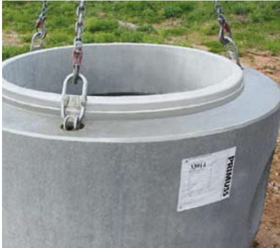
Fig. 3 Label on the completed manhole base.
