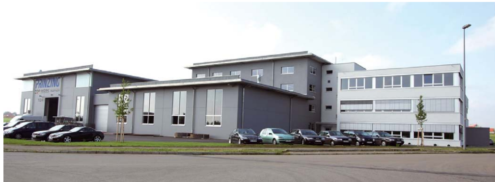
The new company building offers a floor space of 5000 m 2
